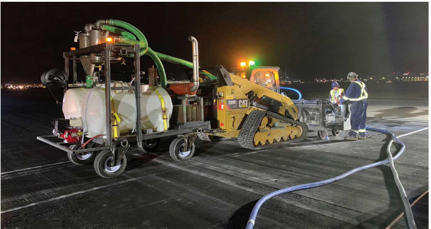
1st totally self contained, saw, skid steer and vacuum in action
