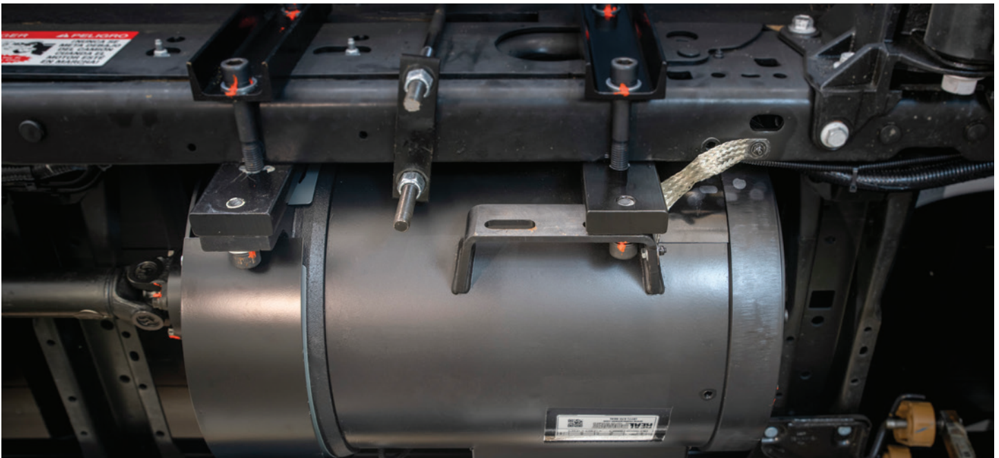
Example of a ground strap connecting a vehicle generator to the frame for system grounding per 250.34 (B) (1)
