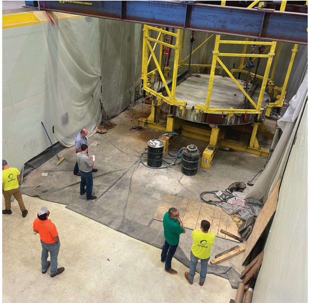
Final MPRV Platform and Pulley Supports In-Place Over Reactor Vessel Mock-Up
