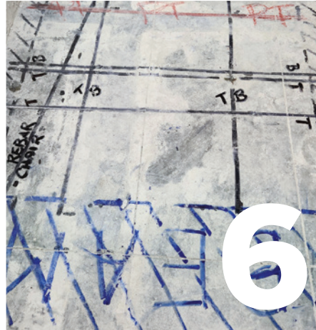
Scanning for Success on a $100M Wisconsin Casino Renovation
