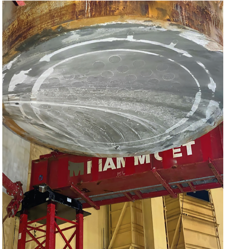
View of First Horizontal Cut - Looking at Bottom of Upper Section of Reactor Vessel
