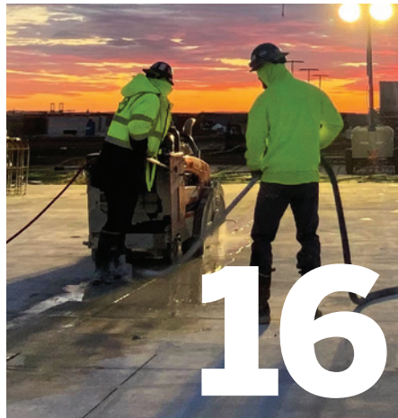
Concrete Parking Structure Safely Demolished with Diamond Tools
